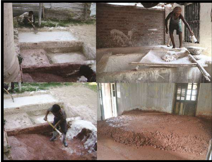
Figure 6. Use of lime mortar during restoration of heritage building
