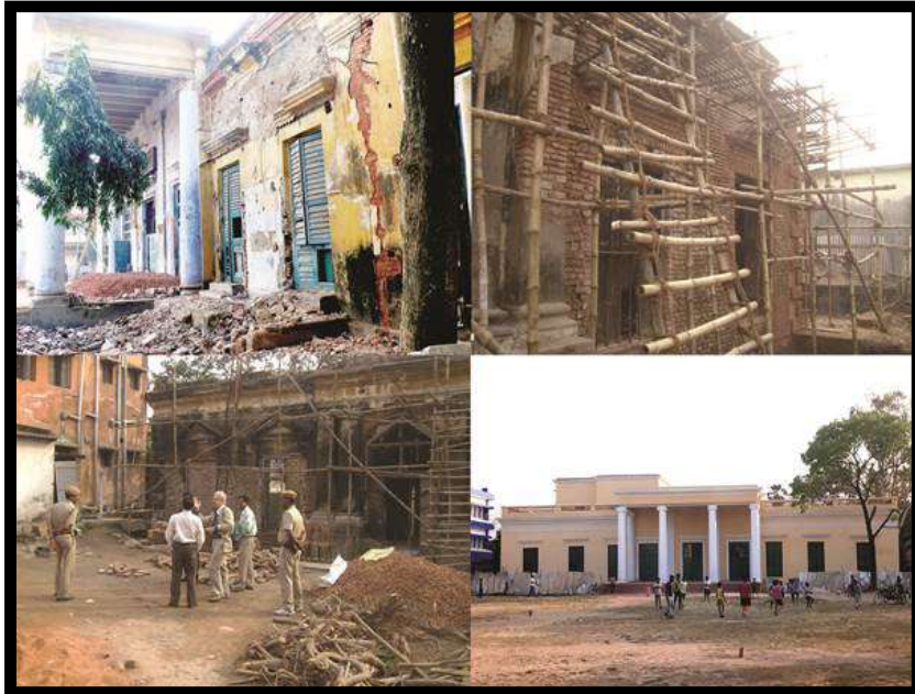
Figure 1. Danish Governor House, Serampore – a restoration project of WBHC
